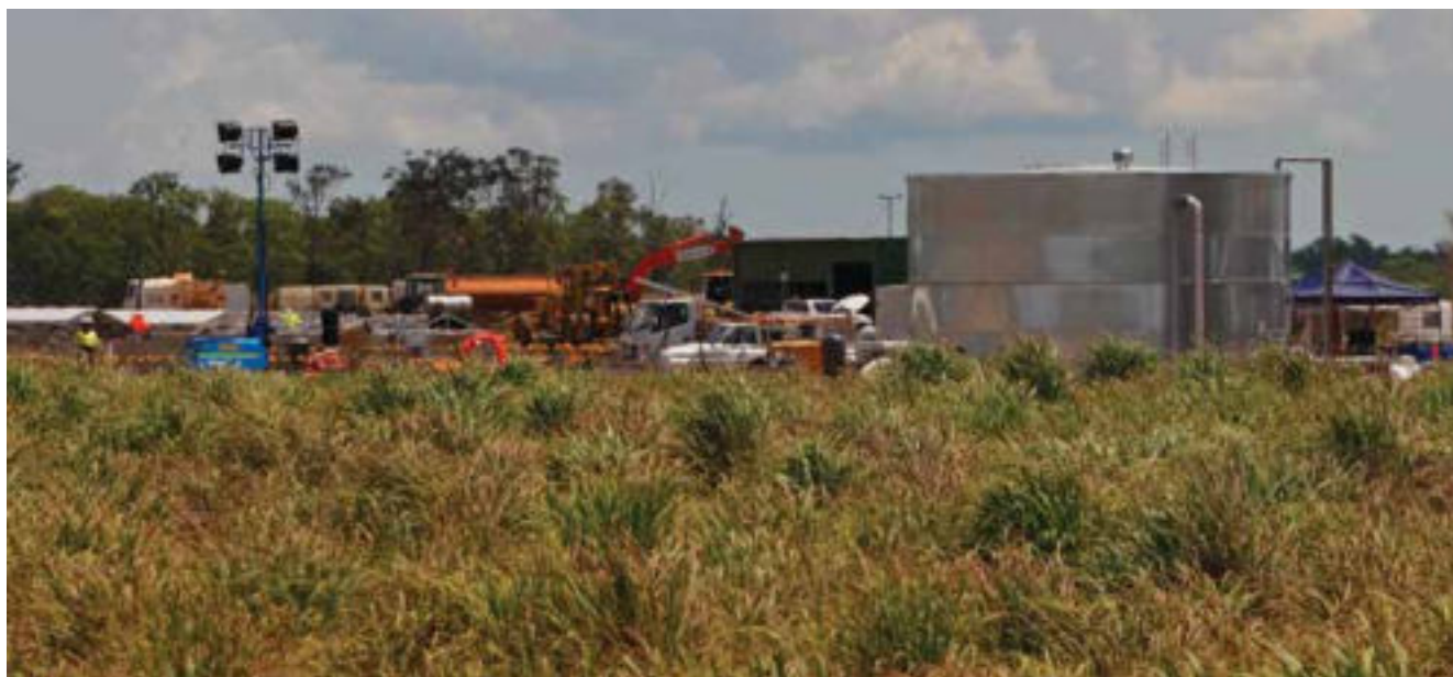
Image: Construction of the new crocodile farm at Lambells Lagoon, Northern Territory.
